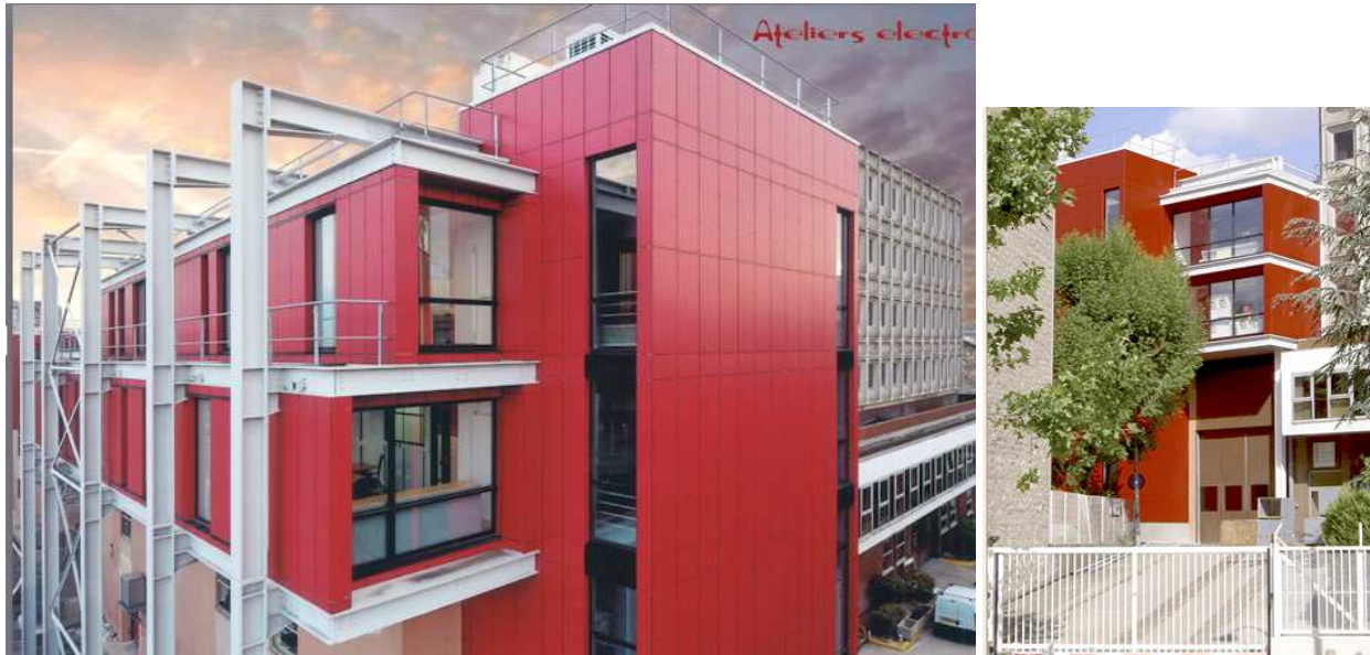
View from the corner of workshops - view of access
