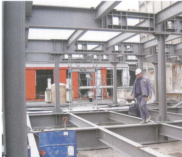
View of main steel frame on site
