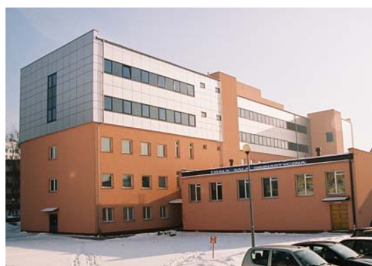
Renovated building showing its 2 new floors
