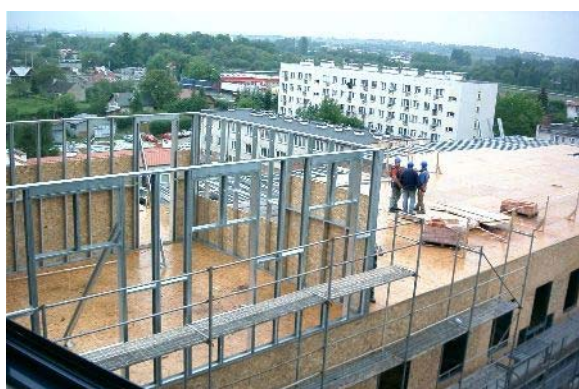
Roof-top extension during construction
