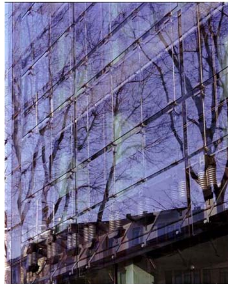
Outer glass facade
