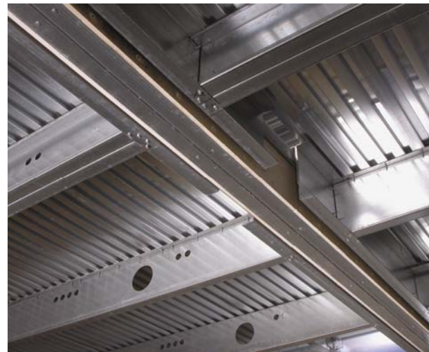
Light steel floor joists
