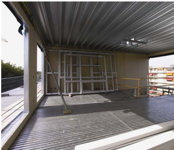
Roof-top extension during construction
