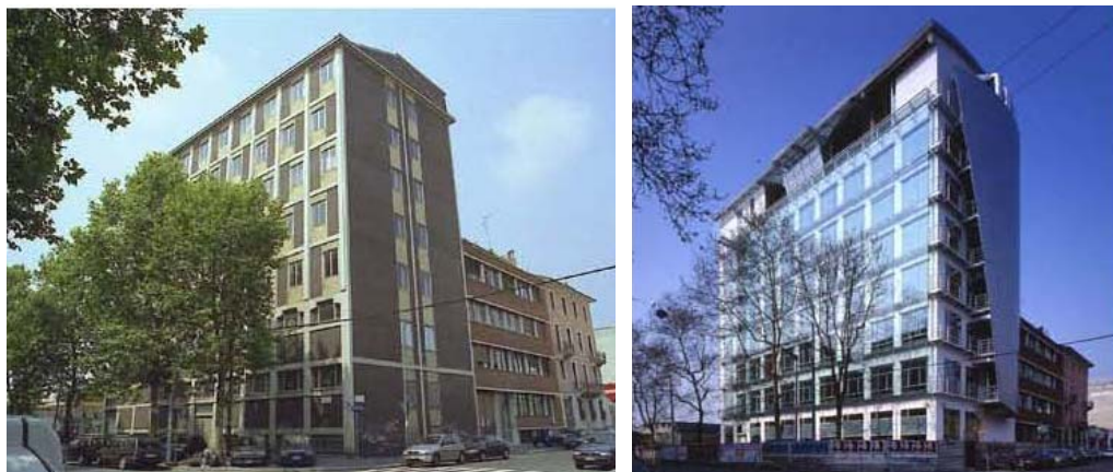
building before and after renovation
