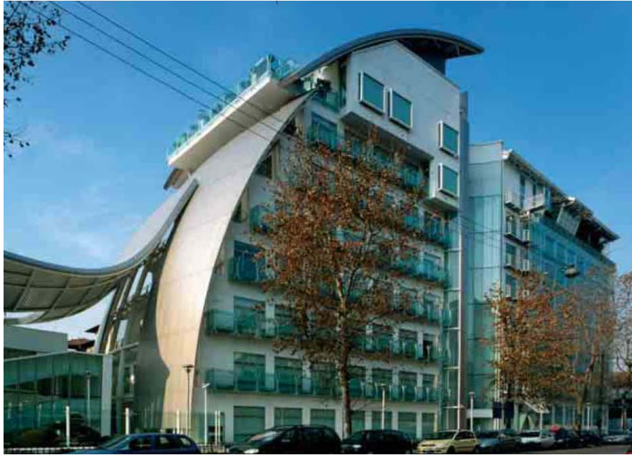
Overall view of Torno Internazionale
