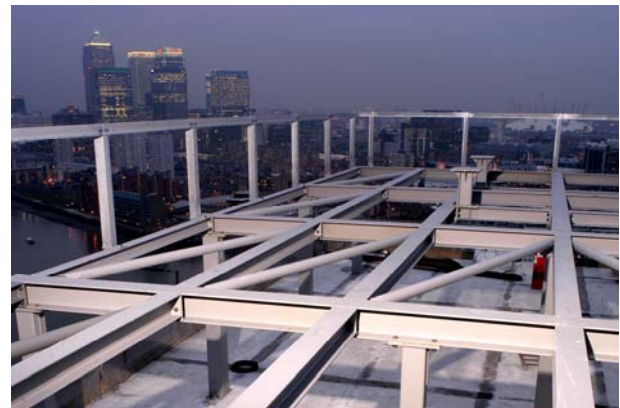
New steelwork at roof level
