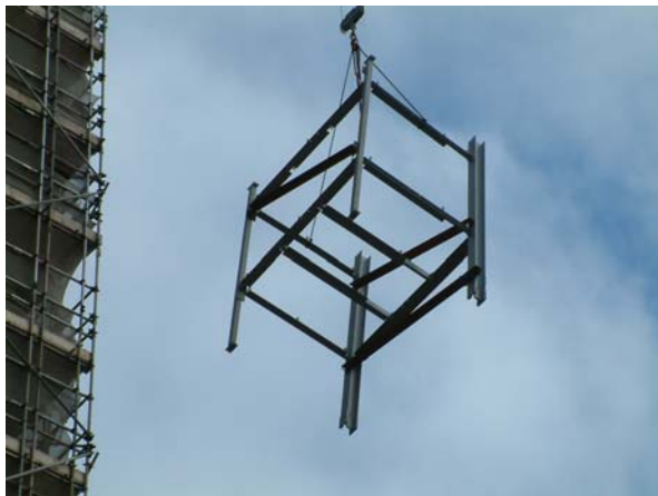
Installation of pre-fabricated steel frame
