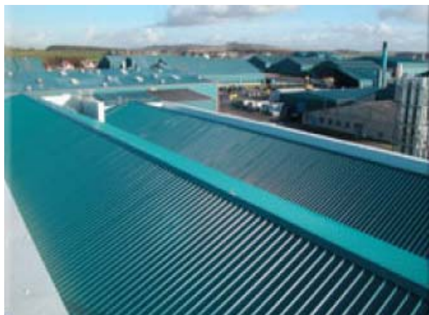
After renovation roof
