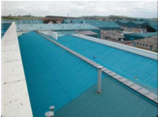
Before renovation of roof roof
