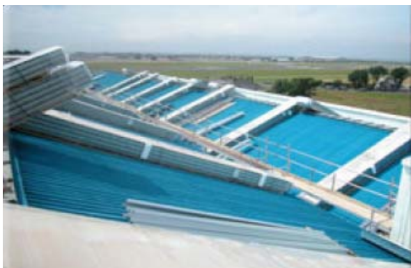
Stock of new purlins stack on the existing roof
