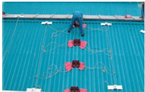
Hole cut through the roof and new cleat connected
