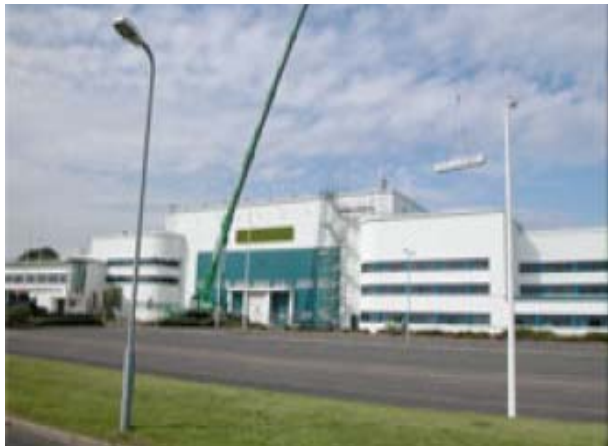
Steel rails support craned on top of
