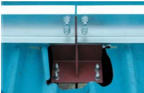
New purlins connected to the cleat
