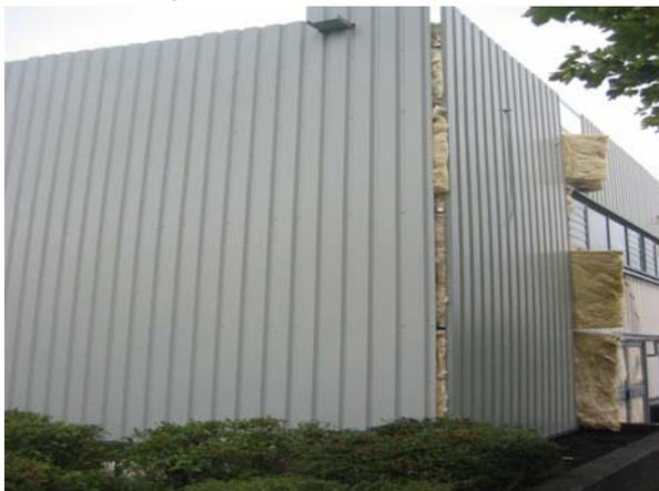
Outer steel profile attached to the existing cladding
