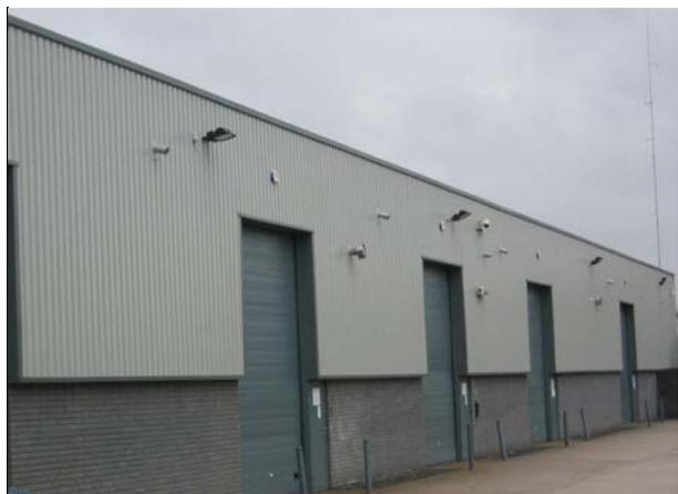
The building is located in central England and is one of the eight buildings currently over-cladded. The work involved the installation of 16, 000m<sup>2</sup> of over-roofing and over-cladding of an existing roof cladding on a building in Milton Keynes, UK using build up system.
