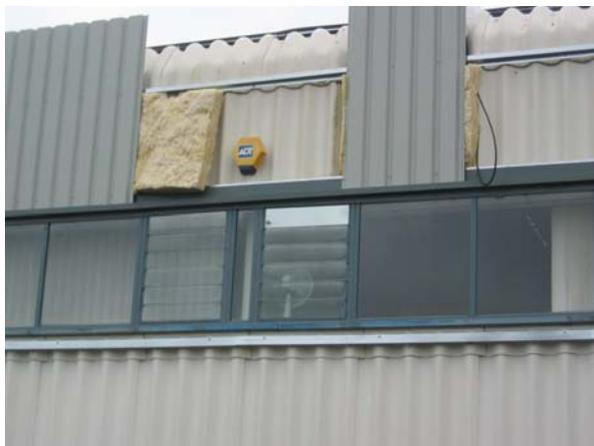
New rail and brackets attached on the existing wall cladding
