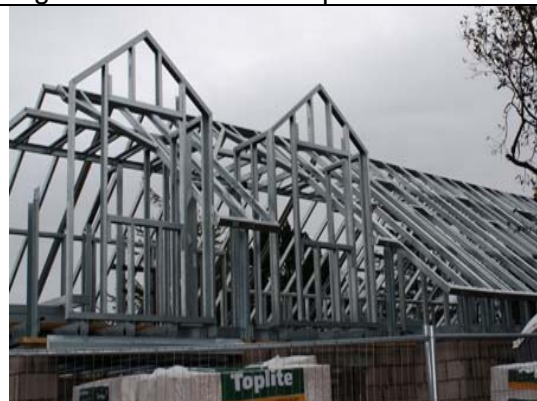
Figure 36: Habitable roof construction phase
