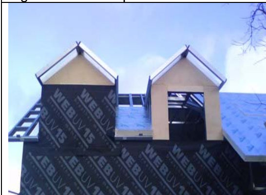
Figure 35: Attic Truss for habitable roof
