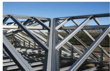
Flat to room in the roof conversion using lightweight steel
