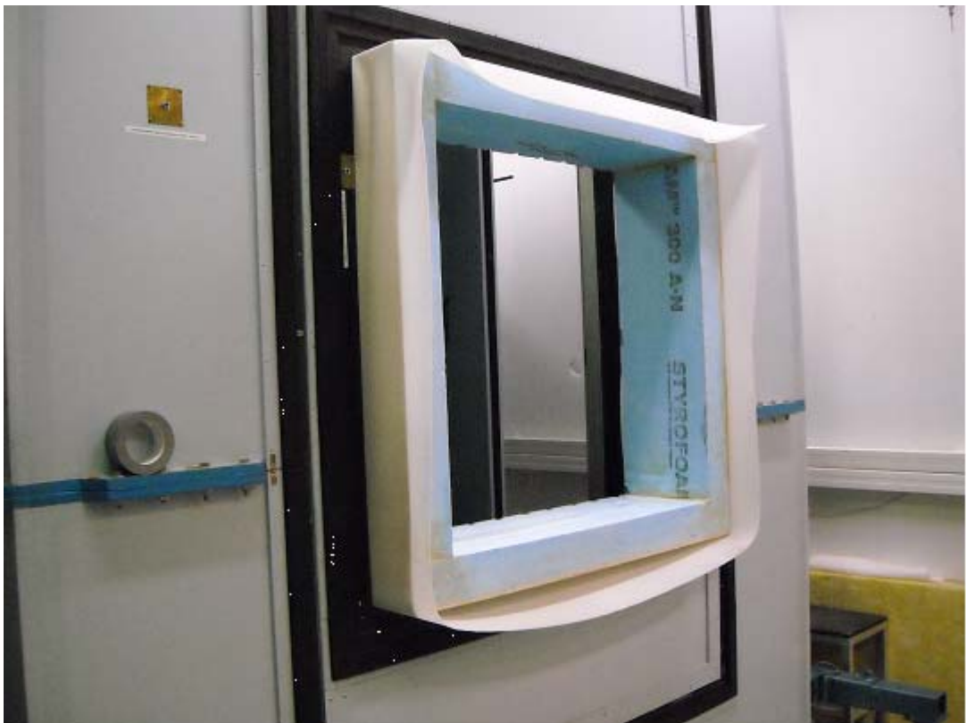
Figure 7. The frame was installed in the test cell facade.
