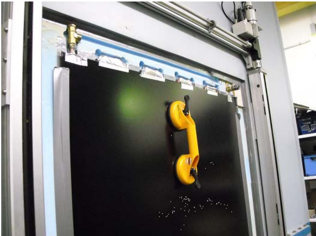
Figure 11. External metal sheet and copper pipes installed in component.
