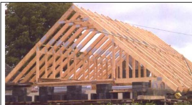
Figure 3: Prefabricated 'Attic Trusses' using timber sections
