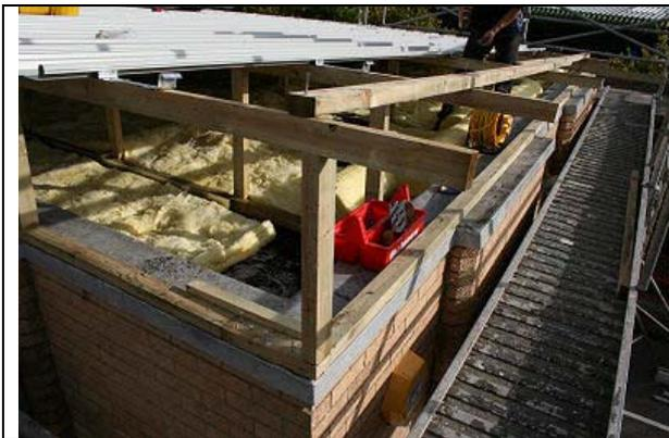
Figure 1: Flat to pitch conversion using timber sections and steel cladding
