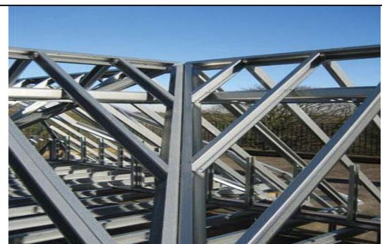
Figure 4: Prefabricated 'Attic Trusses' using lightweight cold form steel sections
