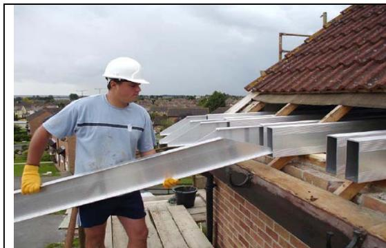
Figure 10: Aluminium I-section and box section installed from the eaves
