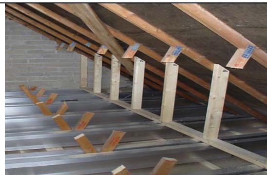
Figure 11: Aluminium floor beams supporting timber cheek wall
