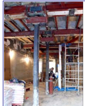
Cast iron column beneath timber beam
