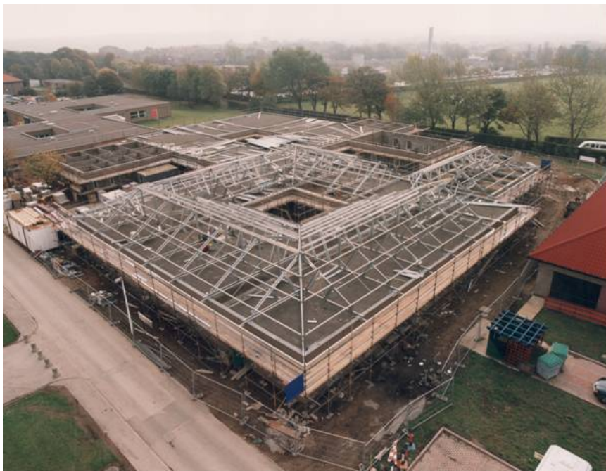
Figure 3 Over-roofing of a single storey hospital building
