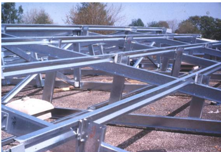
Figure 5 Capella system by Kingspan using light steel C sections
