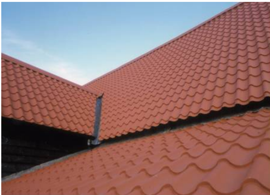
Figure 12 Composite panels with 'roof-tiles' used in refurbishment
