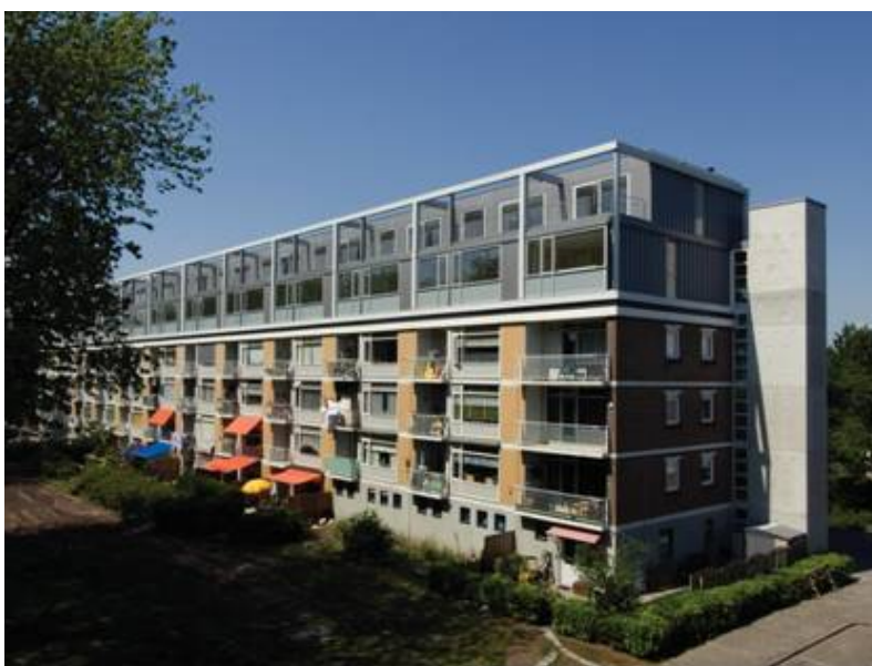
Figure 8 Roof-top extension of a project in Rotterdam
