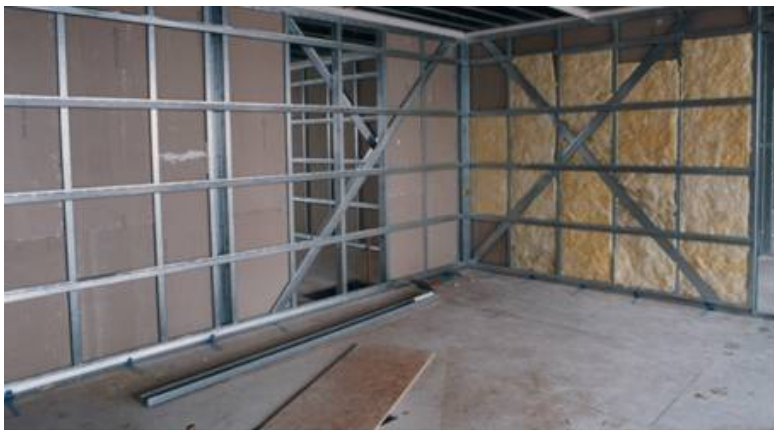
Figure 7 Light steel framing for the new structure in Figure 6
