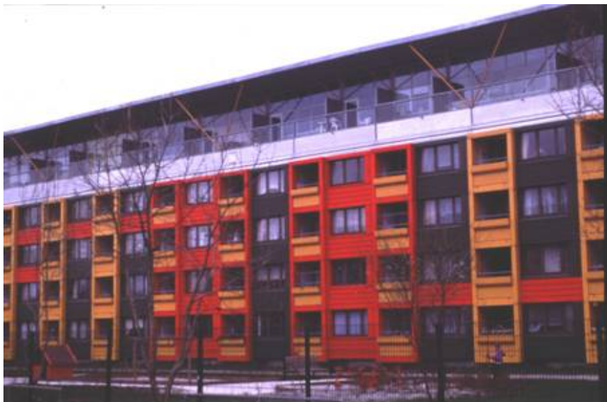
Figure 9 Over-roofing and over-cladding of an existing 4 storey residential building in Denmark
