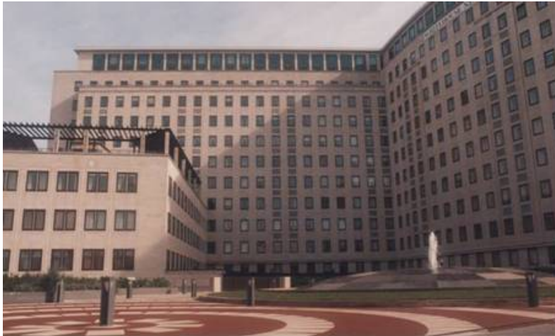
Figure 6 Two storey extension by Metsek to a residential building in London
