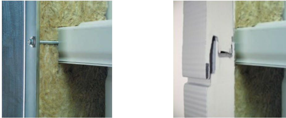
Figure 2: Refurbishment of cassette wall/ built-up-system
