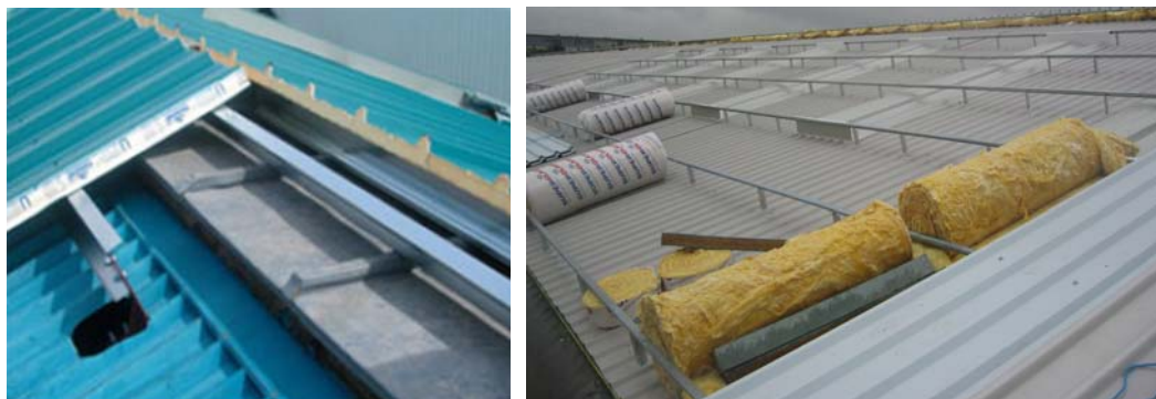
Figure 3: Over-roofing (left), re-cladding (right) for industrial buildings
