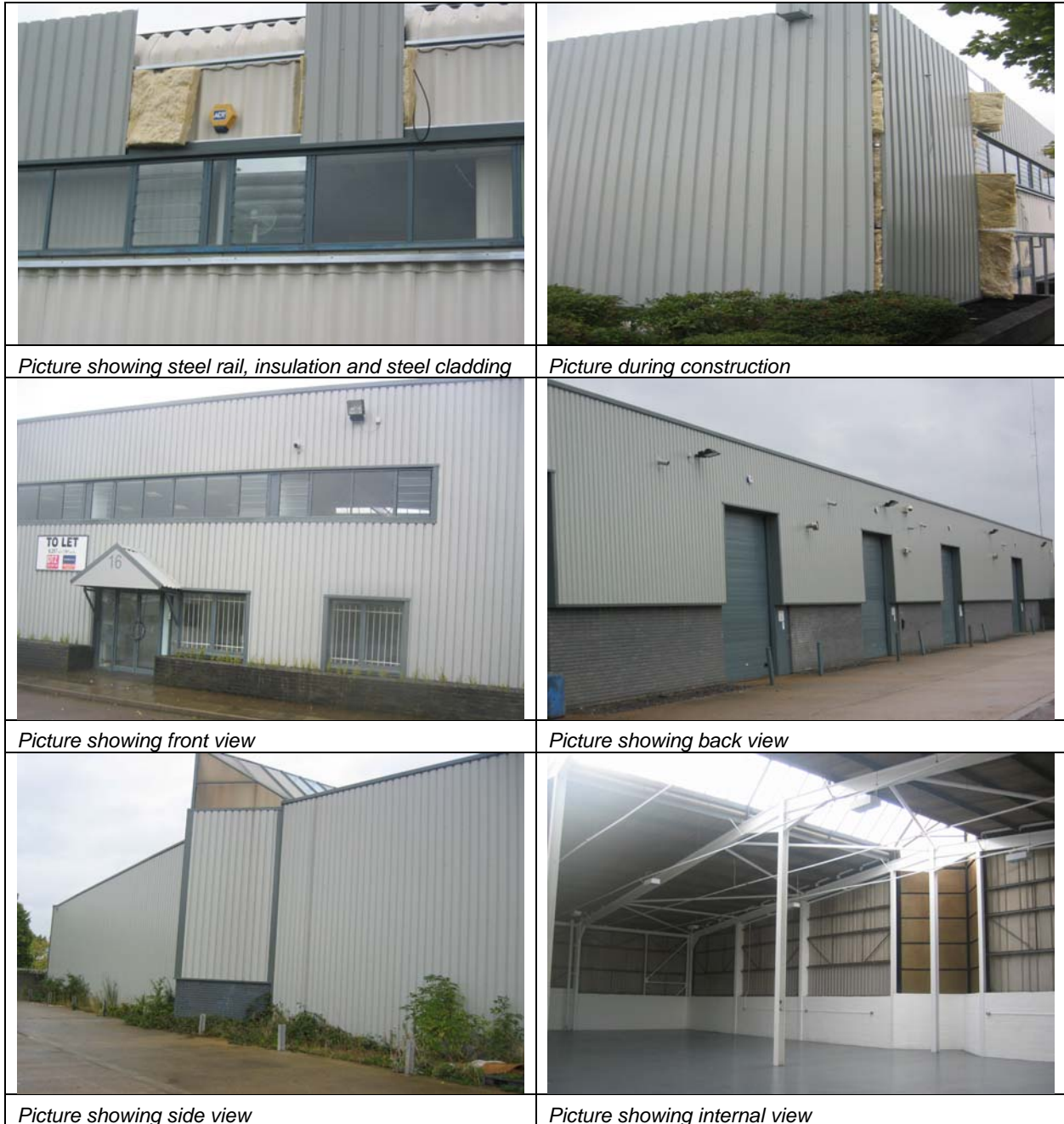
Figure 3: Pictures showing unit 16
