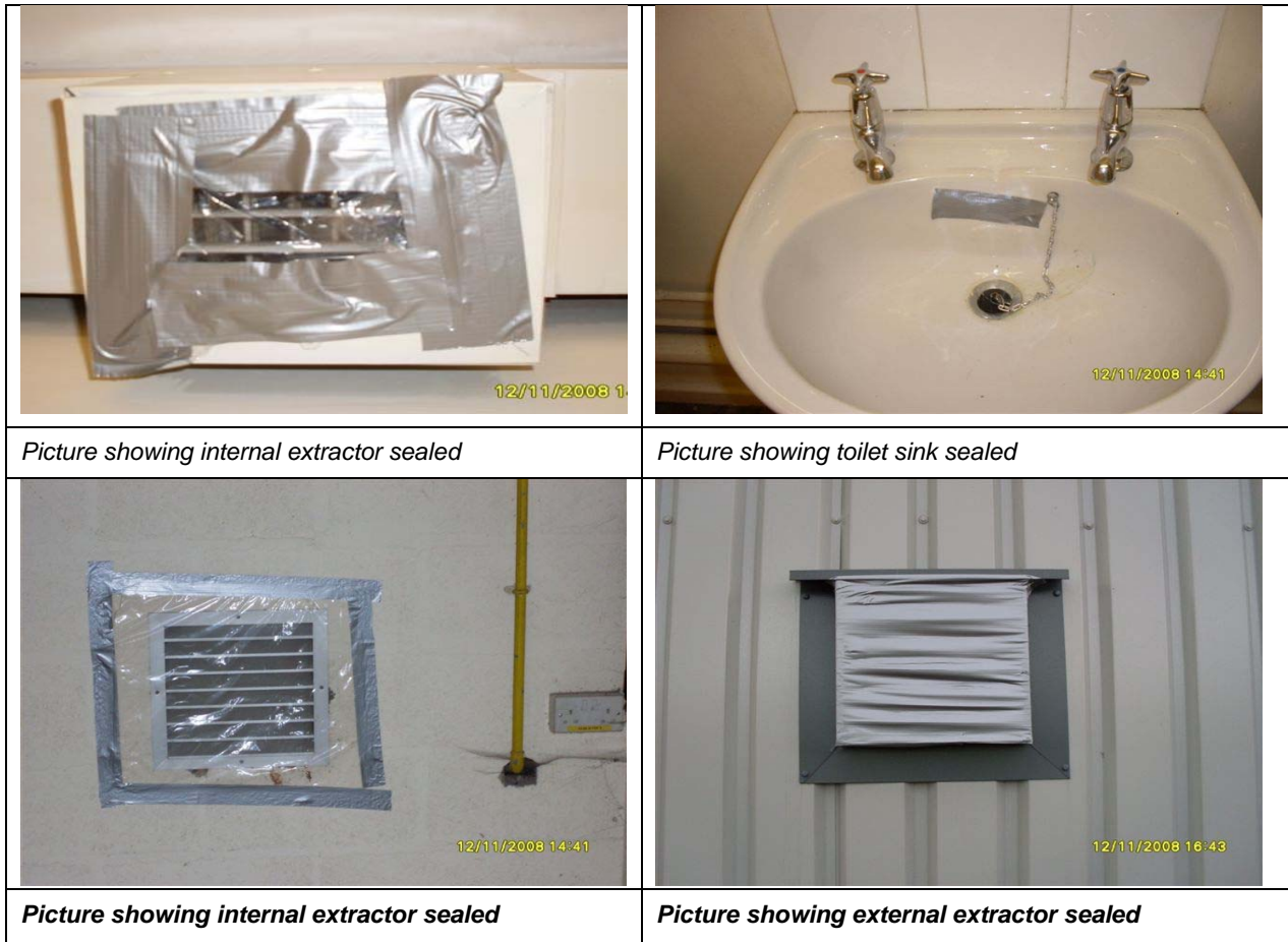
Figure 4: Picture showing temporary sealing for the test
