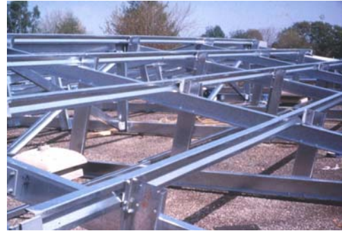
Over-roofing with steel trusses
