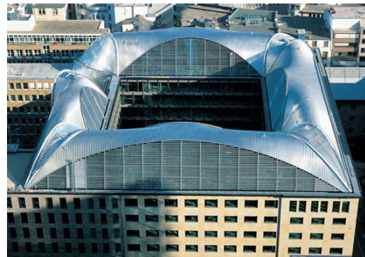
Over-roofing of German Sports Hall
