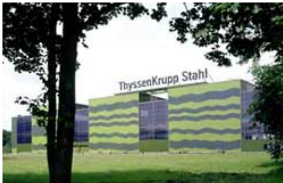
Over-cladding of Industrial Building, Duisburg
