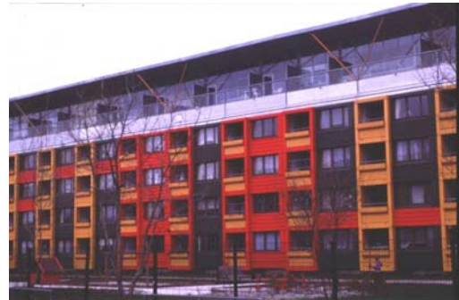
Roof-top extension and over-cladding, Copenhagen
