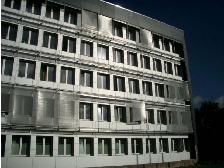
Fig. 10: External solar shading in stainless steel (GKD, Düren)
