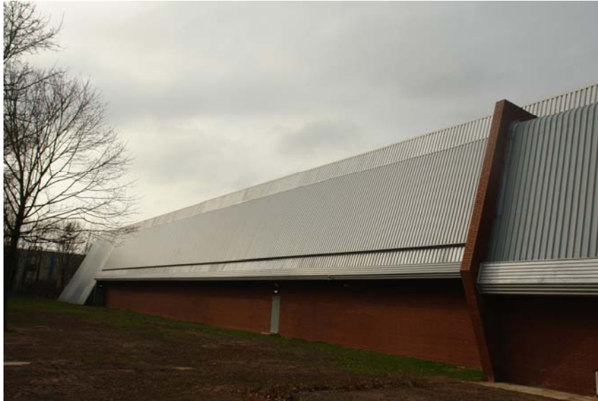
Figure 3 Typical SolarWall ® building in Leamington Spa , UK
