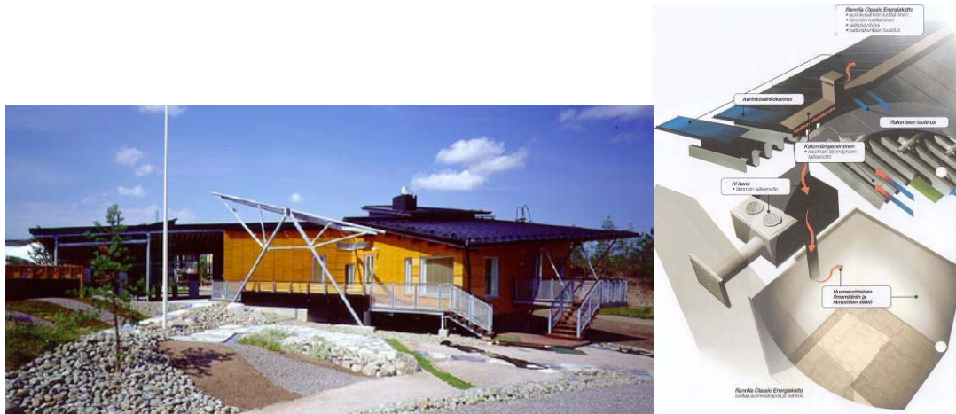
Figure 5 Ruukki demonstration building in Tuusuula, Finland
