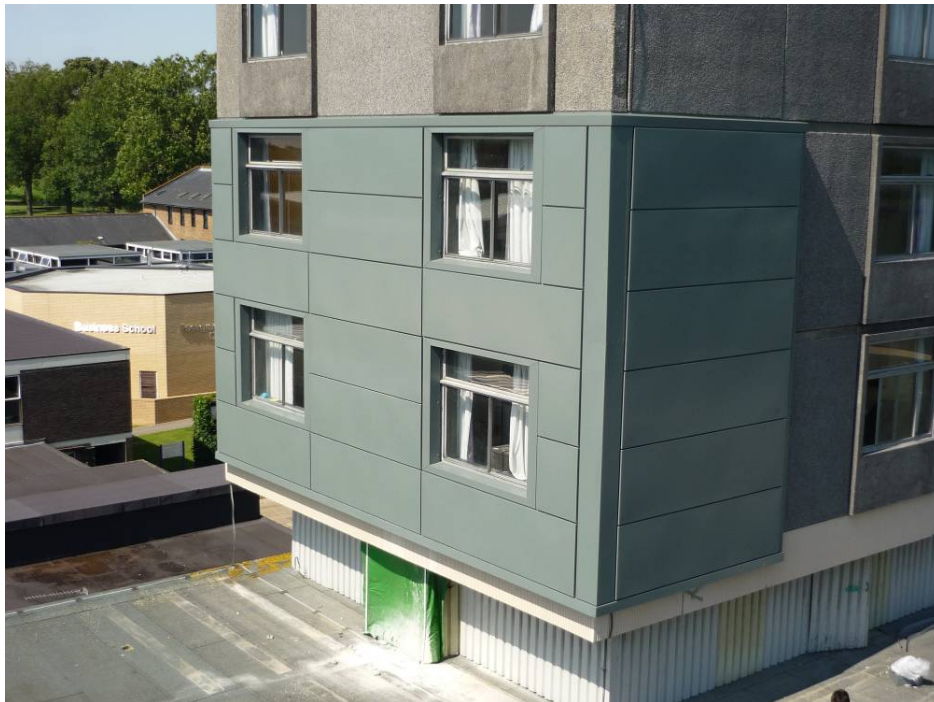
Figure 11 Completed over-clad façade (19 August 2009)
