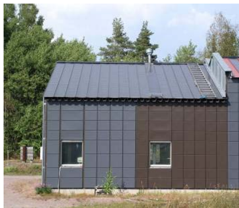
VTT's test roof. The roof slope is approximately 30°, facing south
