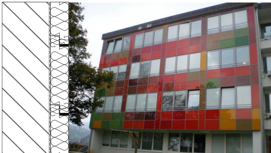
Figure 9: Panel system and application in High-quality passive house renovation in Weiz (Austria)
